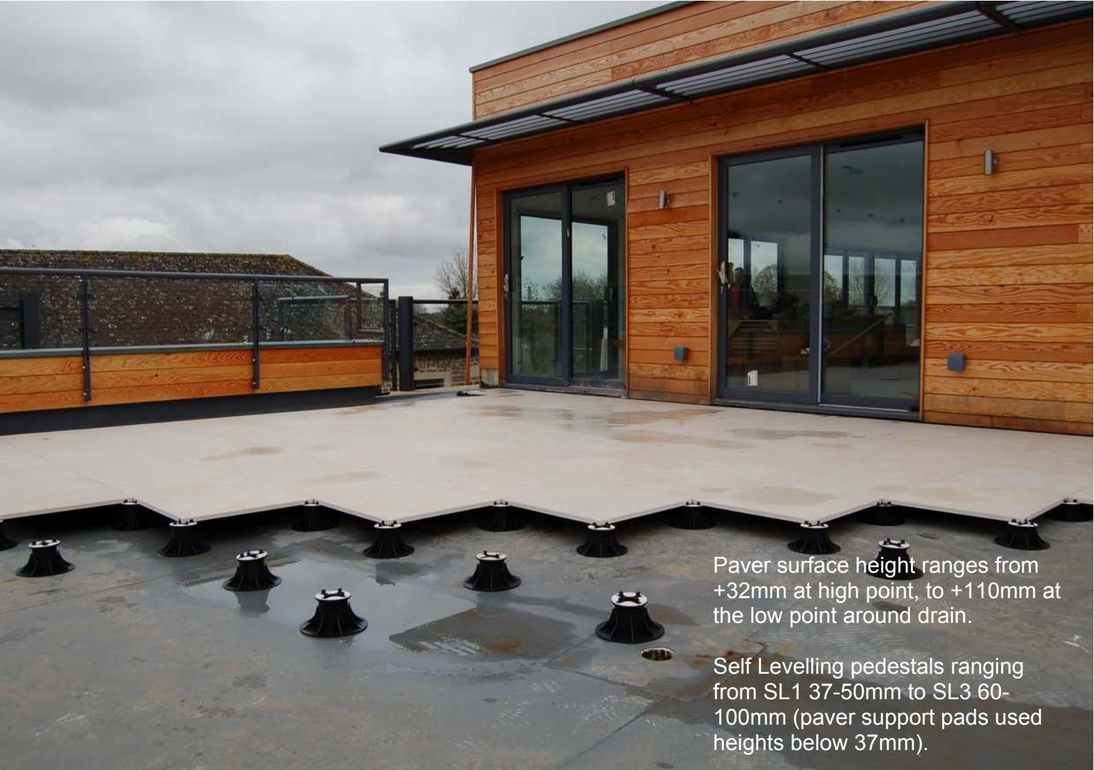
Paver surface height ranges from +32mm at high point, to +110mm at the low point around drain.
